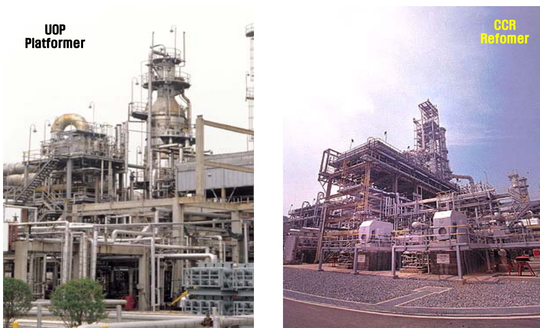
<사진 3-3> Naphtha Hydro-treating unit & reformer unit
